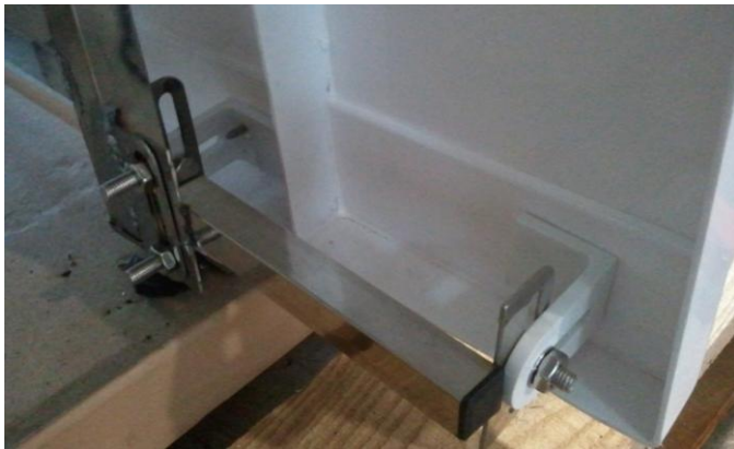
Attaching bottom brackets:
